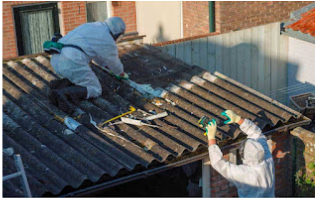
Asbestos Garage Roof Removal And Replacement www.asbestosgarageroof.co.uk
